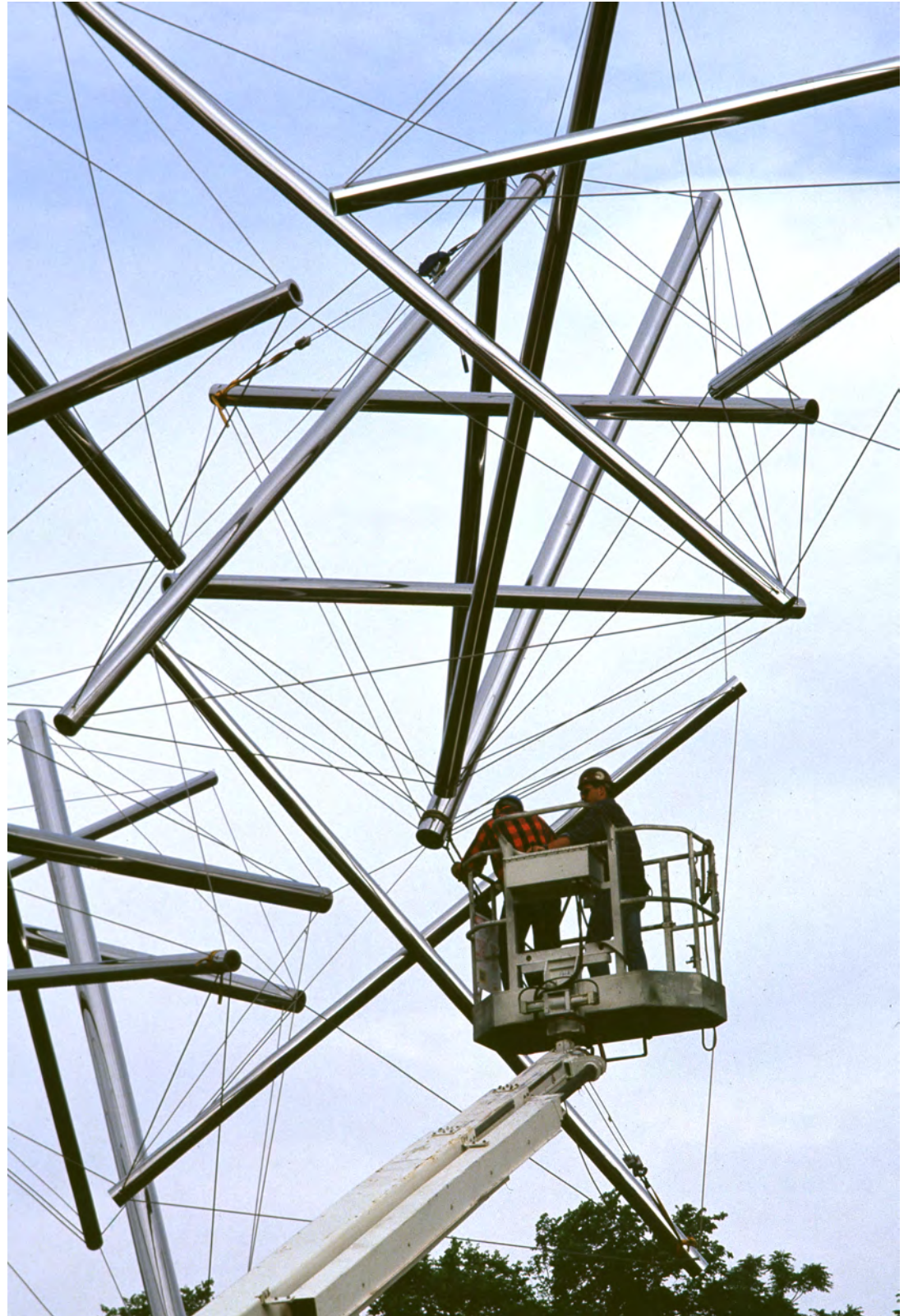
Triple Crown Installation, Crown Center Kansas City MO 1989
