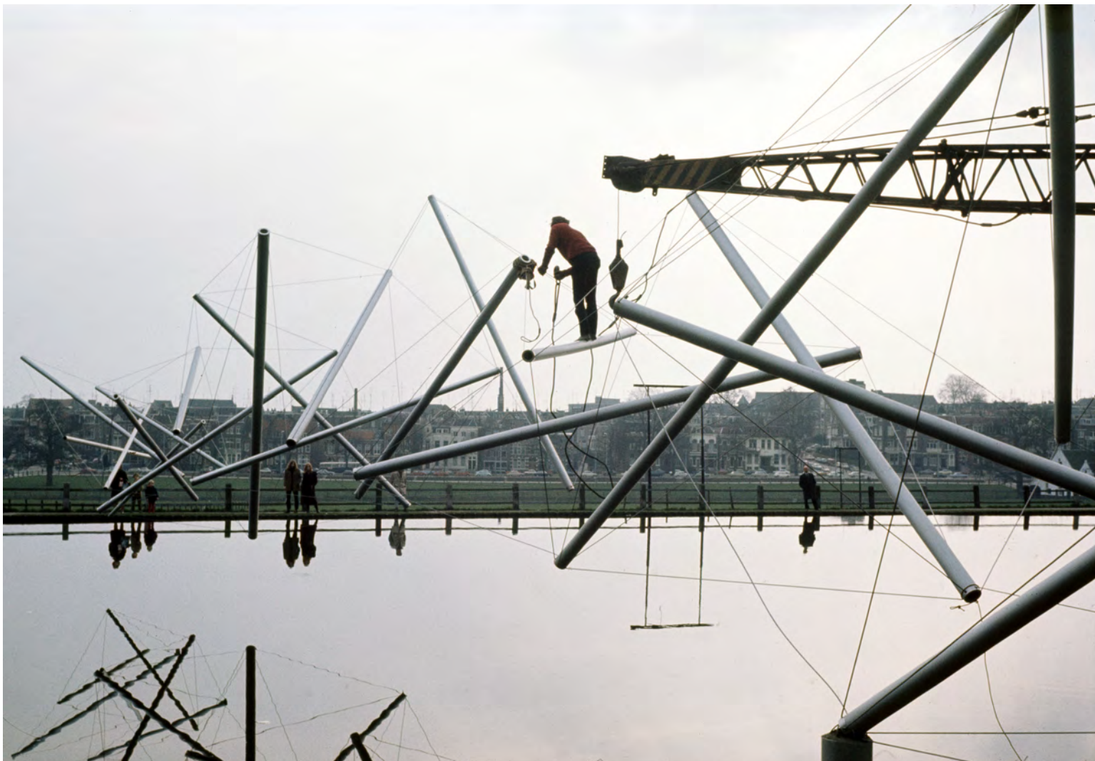
Assembling and installing Easy-K , Park Sonsbeek
