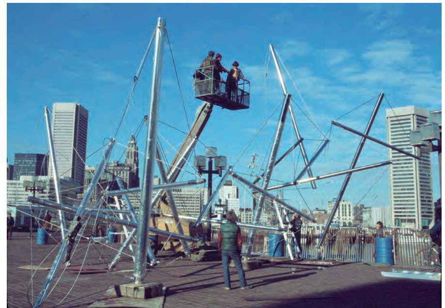
Installing Easy Landing , 1977, Baltimore, MD
