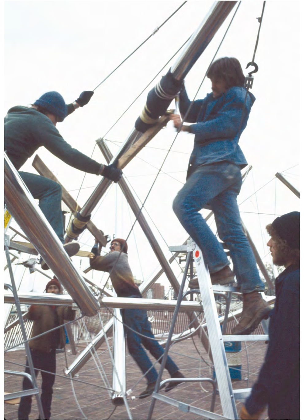
Installation of Easy Landing Baltimore Inner Harbor, MD, 1977
